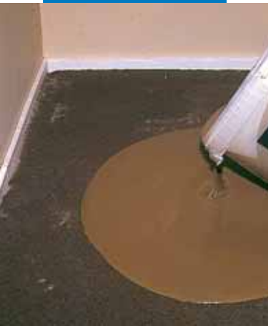
Applying the Novoplan 21 paste on the substrate
