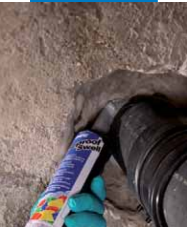
Through element sealed using Mapeproof Swell
