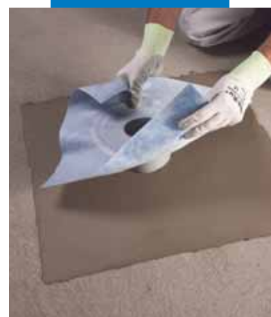
Application of Drain Vertical on Mapelastic
