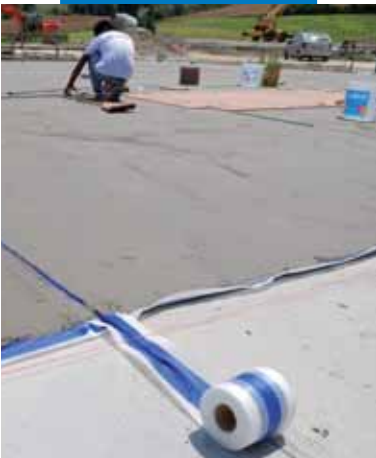
Waterproofing screeds with Mapelastic and Mapeband
