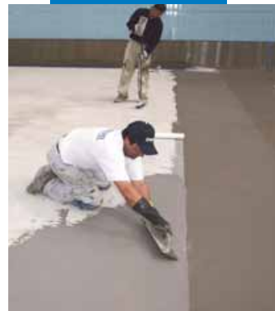
Waterproofing a swimming pool with Mapelastic
