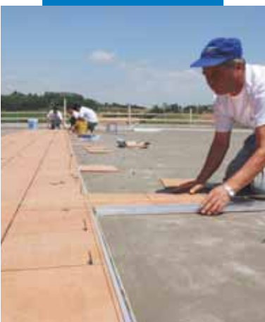
Installing ceramic with Kerabond + Isolastic
