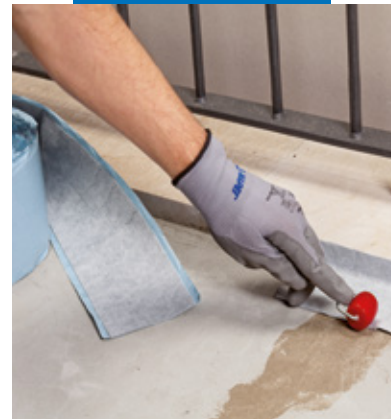
Application of Mapeband SA around edges
