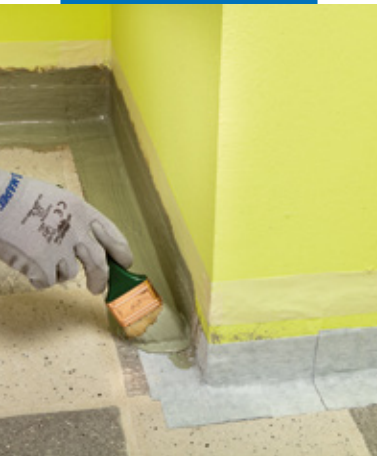
Application of Mapeband SA on a screed
