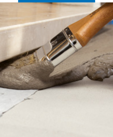
Application of Mapeband SA in difficult areas, such as under a doorstep
