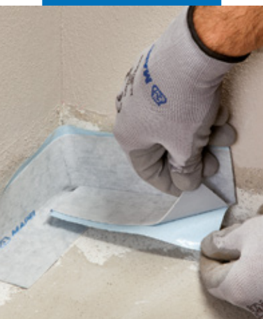
Application of Mapeband SA in corners
