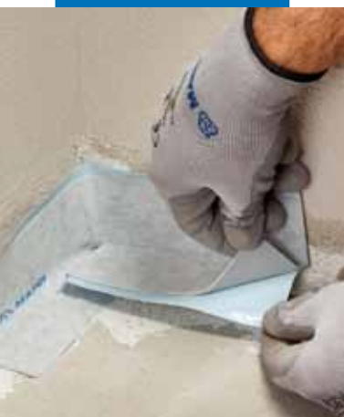
Application of Mapeband SA in corners
