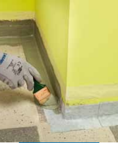
Application of Mapeband SA on a screed
