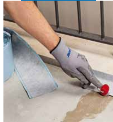
Application of Mapeband SA around edges
