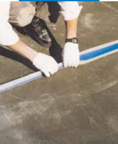
An example of waterproofing an expansion joint on a terrace
