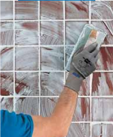
Laying the product with a rubber float
