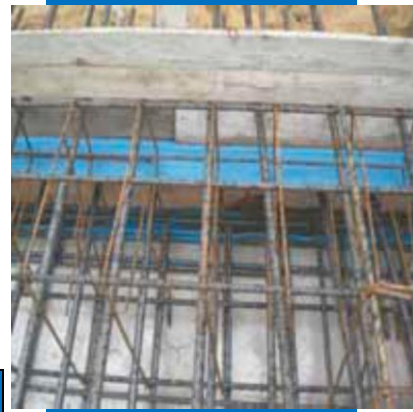
Sealing a structural joint on foundation
