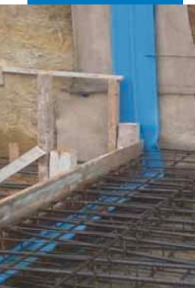
Sealing a structural joint on a vertical wall
