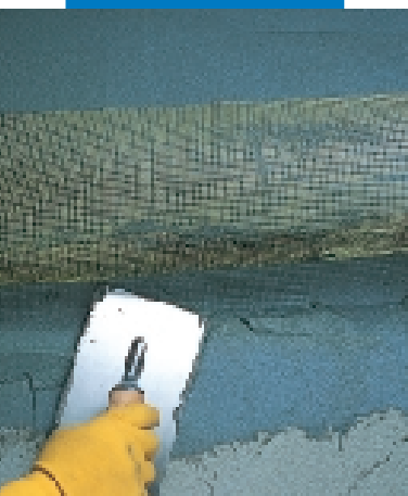
Waterproofing with Mapelastik reinforced with Fibreglass mesh
